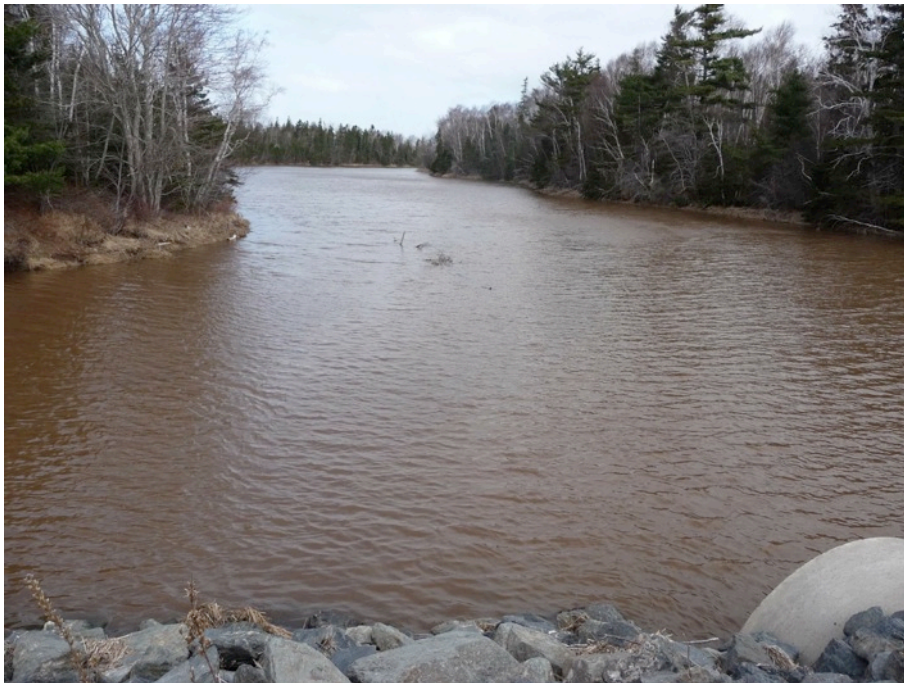
Figure 2 Downstream of Smith Gut causeway at high tide.
