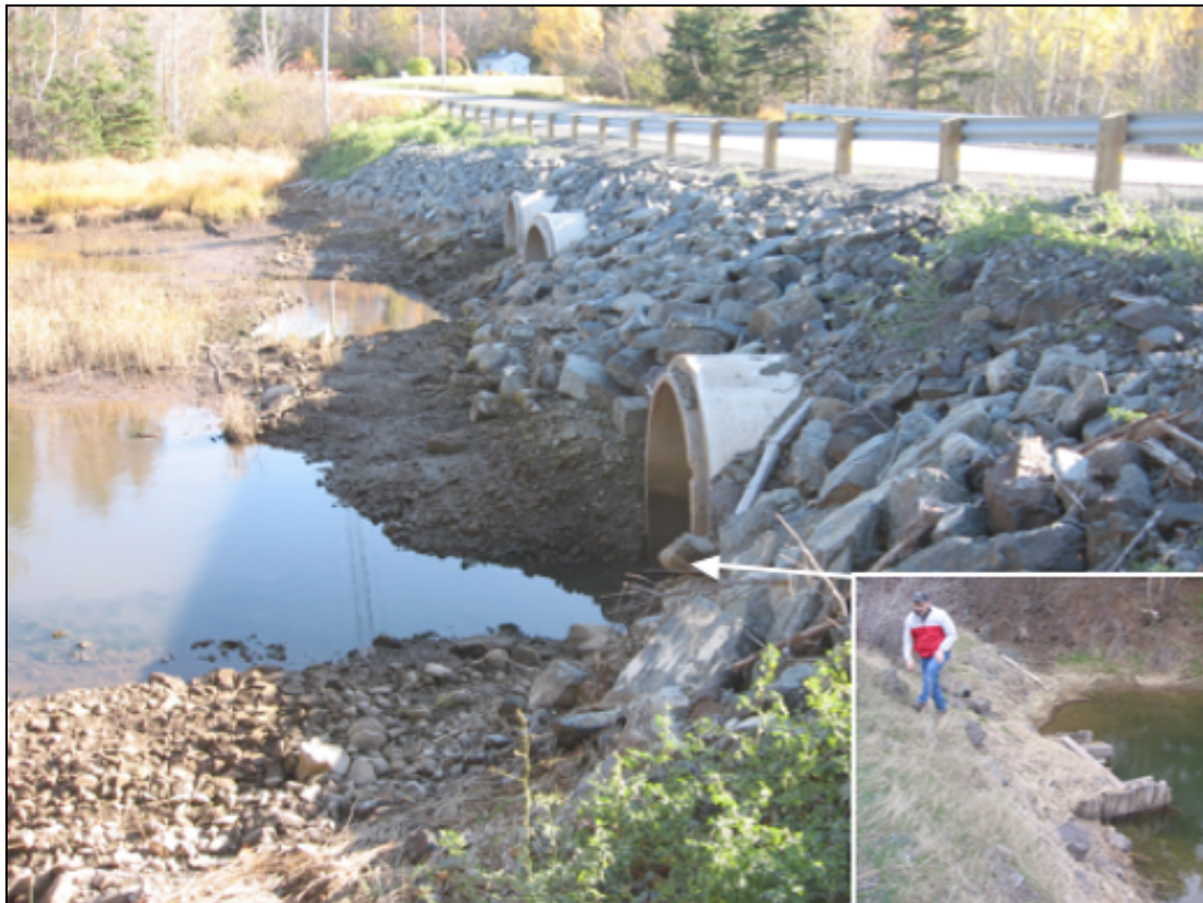
Figure 5 The three concrete culverts installed at SG in 2006 (downstream). Photograph was taken at low tide, when water only flows through one of the three structures (culvert in the foreground). Photograph by T. Bowron, 2007. The inserted picture is of the original culvert, taken 2 May 2006, courtesy of Dr. Bob Pett.
