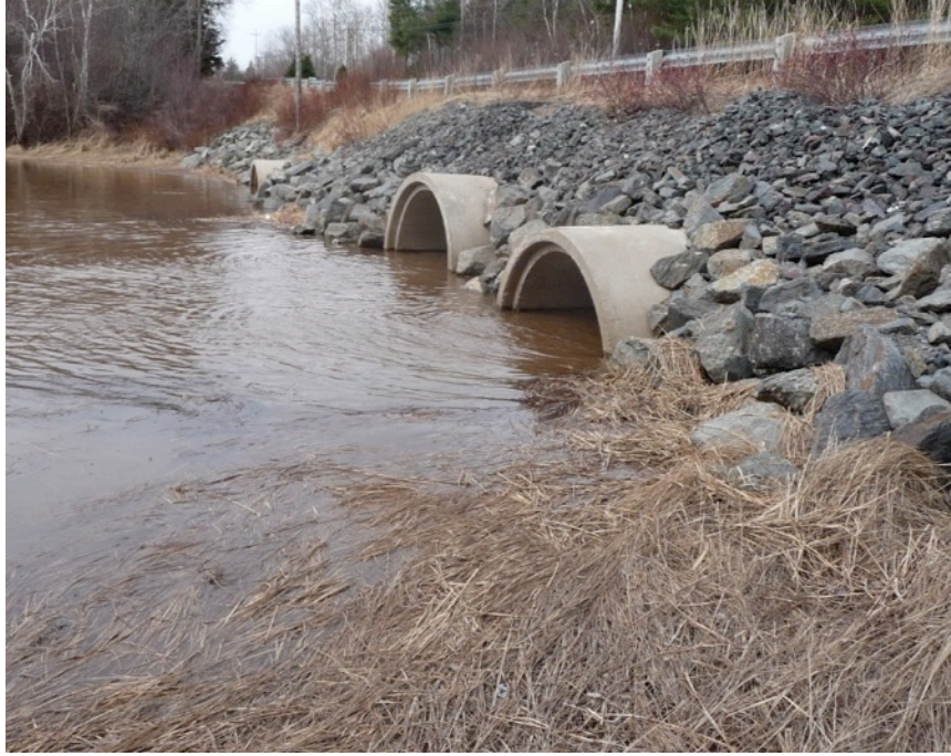
Figure 1 Culverts from upstream side of causeway at high tide.
