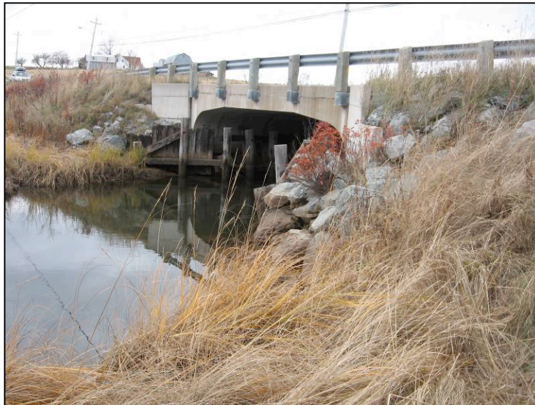
Figure 8 Huggans Brook causeway-bridge tidal crossing. Photograph by T. Bowron, 2007.
